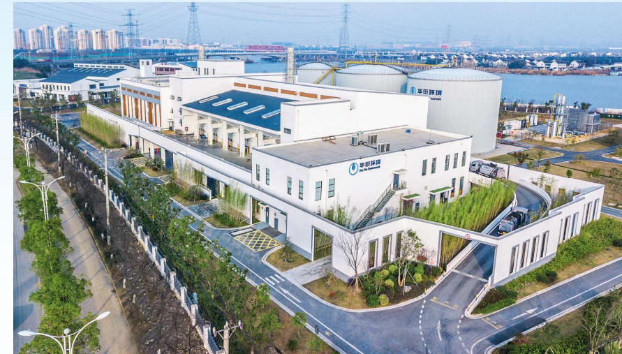
Suzhou Food Waste Treatment Project
