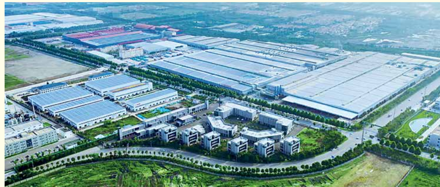
集團於江蘇省徐州市賈汪工業園區以蒸氣代替煤，為區內企業及居民供應熱能。 At Jiawang Industrial Park in Xuzhou, Jiangsu province, we supplied steam heat to local residents and businesses as a replacement for coal.
