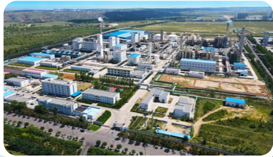
Methanol Plant, Inner Mongolia
