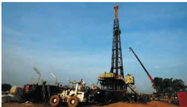
An Onshore Oilfield Exploration Project in Thailand
