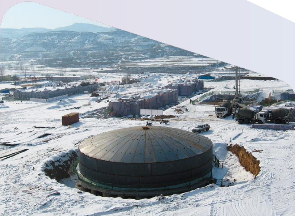
The natural gas liquefaction plant taking shape in Shanxi.
