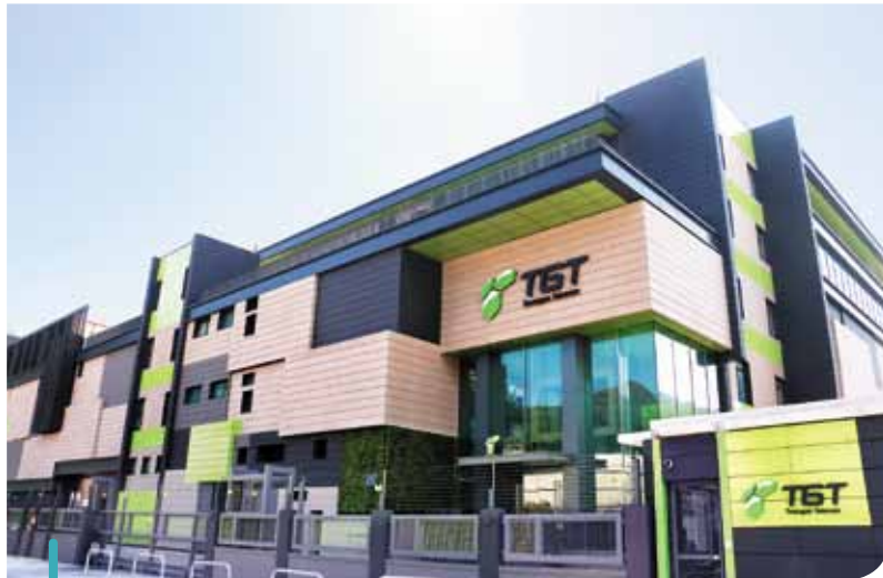
Equipped with TIA-942 Tier 3+ facilities, the TGT Tseung Kwan O Data Centre 2 is fully operational, providing world-class professional services to clients.
