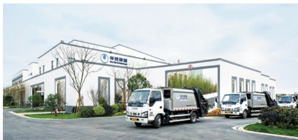
▲ The Group's first food waste treatment project in Suzhou Industrial Park
