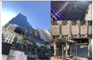
H Zentre on Middle Road in Tsim Sha Tsui utilises solar-powered integrated primary air handling units (Integrated D-PAU) with desiccant wheels. By combining heat energy from solar collectors with gas water heaters, hot water is produced to dry the desiccant wheels and regenerate their dehumidification capacity, thereby effectively reducing energy consumption and improving indoor air quality.
