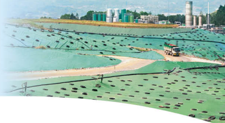
● 公司不斷開拓潔淨能源，圖為新界東北堆填區的沼氣應用項目。 The Company is committed towards the development of clean energy. This photo shows our Northeast New Territories Landfill Gas Utilisation project.
