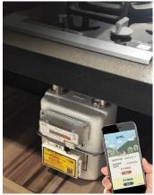
Towngas is actively promoting innovation, such as the development of a new generation of the Towngas Smart Metering System, which connects to a smart meter via WiFi and the "Towngas Metering" mobile app to automatically report the meter reading every month, simplifying the process.
