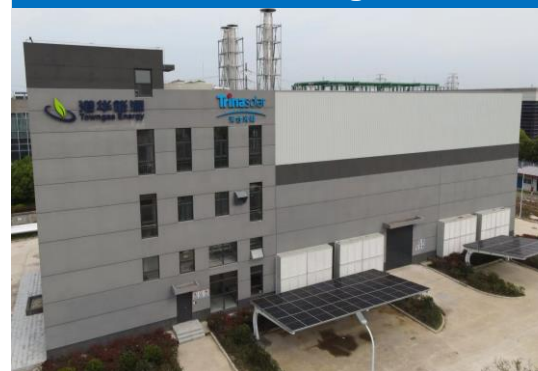
Microgrid Demonstration Project In Jiangsu Province
