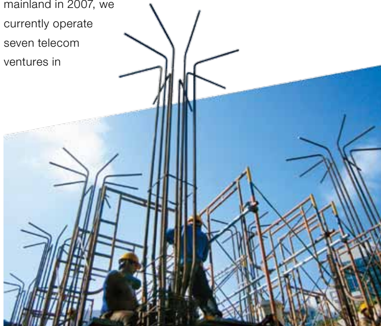
Construction of the Bowen Drive Salt Water Pumping Station, the Magazine Gap Road Salt Water Service Reservoir and associated works by U-Tech for the Water Supplies Department.
