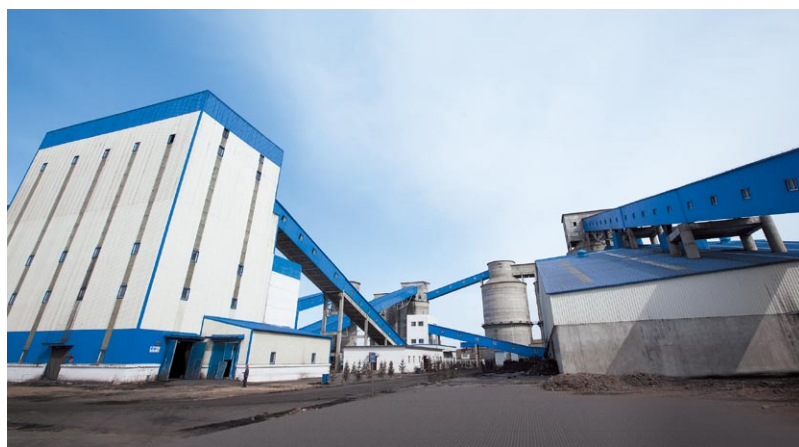
Supplying coal to our methanol plant in the vicinity, the construction of the Xiaoyugou mining facility was completed in Erdos, Inner Mongolia.
