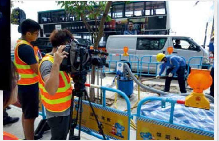
電視台正拍攝「氣動吸泥機」如何有效幫助工人避免長時間彎腰和進行重複性動作。 Pneumatic Soil Remover helps to reduce abnormal posture and repetitive actions of workers.
