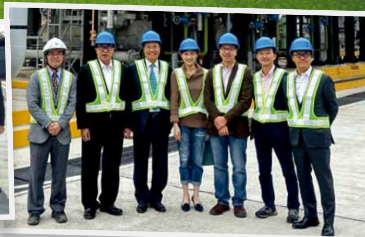
煤氣公司邀請立法會環境事務委員會議員參觀新界東南堆填區沼氣轉化生產設施。 Towngas invited Legislative Council Members of Panel on Environmental Affairs to visit SENT Landfill Gas Conversion Facility.
