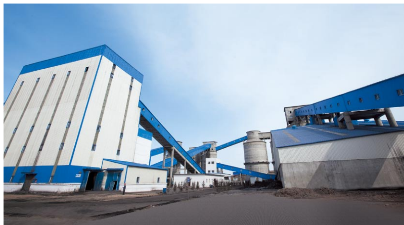
Supplying coal to our methanol plant in the vicinity, the construction of the Xiaoyugou mining facility was completed in Erdos, Inner Mongolia.
