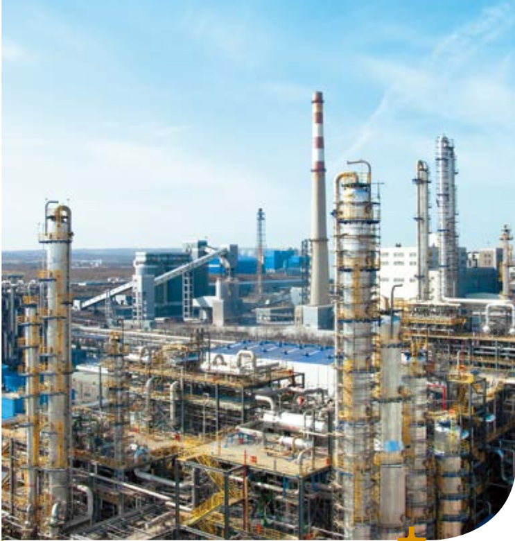
Construction of the ethylene glycol facility in Ordos, Inner Mongolia Autonomous Region, was completed in 2017.
