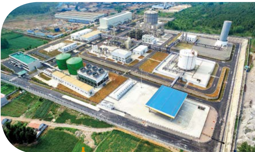
Our coke oven gas plant in Xuzhou, Jiangsu province will commence trial production in the first half of 2018.
