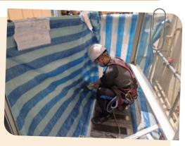
One of these is a dual protection mechanism. It involves the installation of multiple eyebolts and the use of Transportable Temporary Anchor Devices (TTADs) connected to double lanyards to help eliminate falling hazards. Additionally, all workers are required to use hand tools equipped with lanyards to prevent these tools from falling and injuring people underneath.
