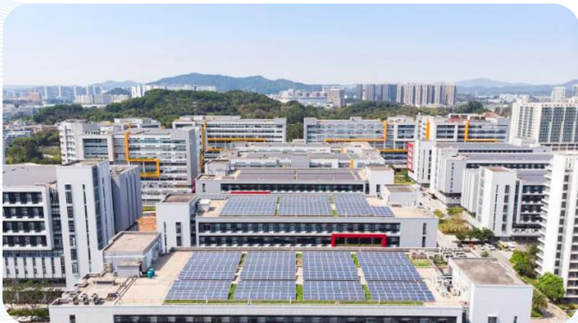
5.5MW distributed photovoltaic power generation project at Foshan Industrial Plant
